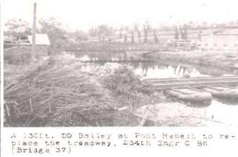
A 130ft. DD Bailey at Pont Hébert to replace the treadway. 234th Engr C Bn (Bridge 37)
